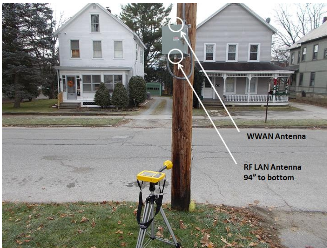
Figure 37. GMP Gatekeeper mounted on a power pole at GMP site 8 with the WWAN antenna on the top and the 900 MHz RF LAN antenna on the bottom.
