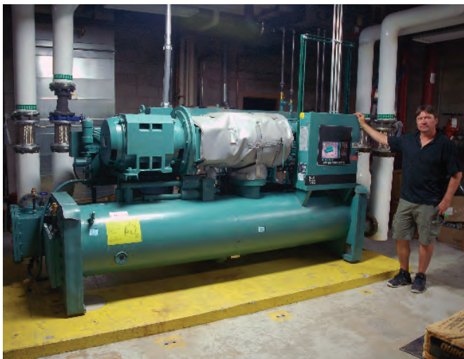
Figure 1: 100-ton water-cooled chiller. Water-cooled chillers use cooling towers to reject heat through evaporation.
